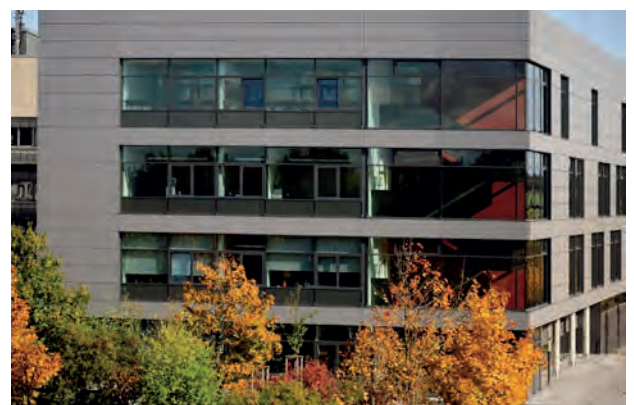
The animal facility – awarded for its architecture. HZI/Schughart
