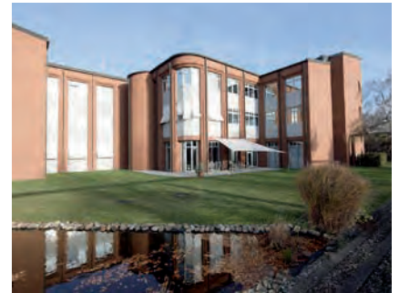
The TWINCORE facilities in Hannover TWINCORE
